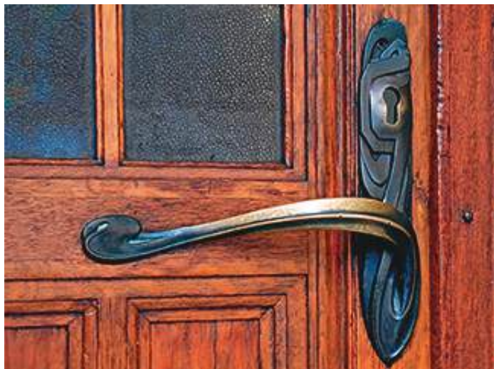
Door handle for the Rue de Florence entrance, designed by Henry van de Velde. Photo Maud Rochez, 2017.
