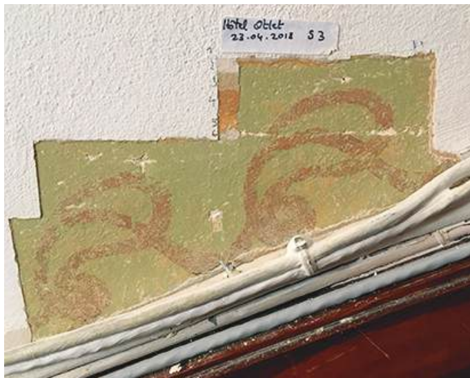
Stratigraphic study in the staircase. IRPA, 2018.13755.
