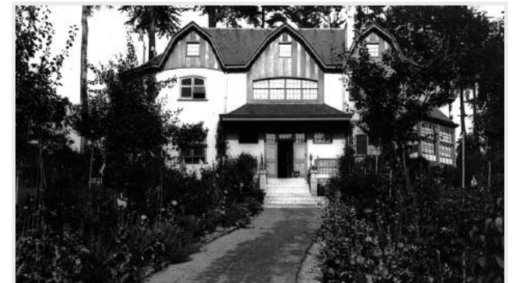
The main façade of the Bloemenwerf with its three different gables. Photo Charles Lefébure, 1899. AML, FS X 882.
