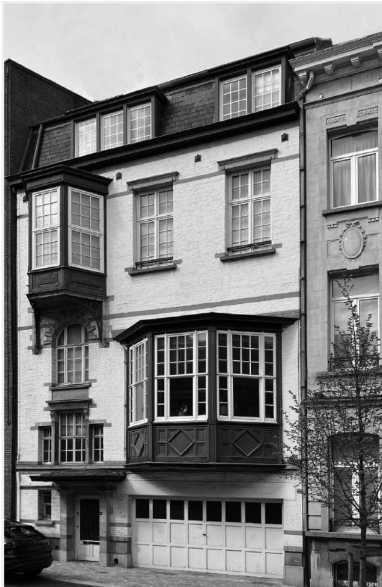
Théo Van Rysselberghe's studio house, designed by his brother Octave, 63 Rue de l'Abbaye at Ixelles [1891-94]. On the ground floor, a garage replaces the previous dining room. Photo Michel Louis, 2024.
