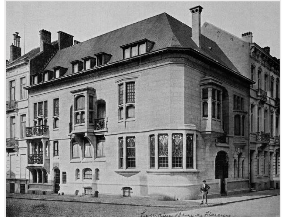
Hôtel Otlet, on the corner of Rue de Florence and Rue de Livourne at Brussels [1900]. CIVA Collections, Brussels, Otlet-R76-0-04.
